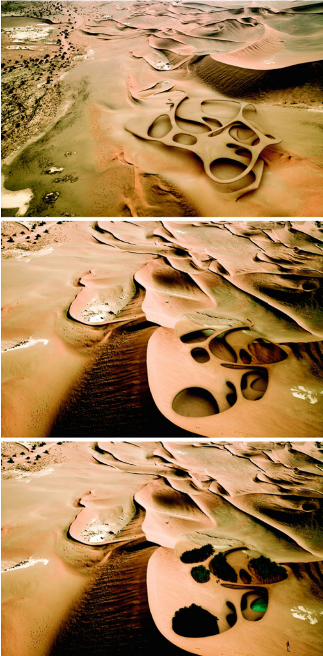
Fig. 4 Pneumatic balloon precipitation: The microbial solution is distributed through specifically designed apertures in the skin of the structure, solidifying the sand surrounding it into structural compressive surfaces
